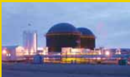
The completed IMUS plant.
